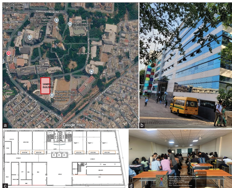
Figure 1: Details of the surveyed reference academic building. (a) Site plan; (b) view of the building elevation, (c) typical floor plan, and (d) classroom view
